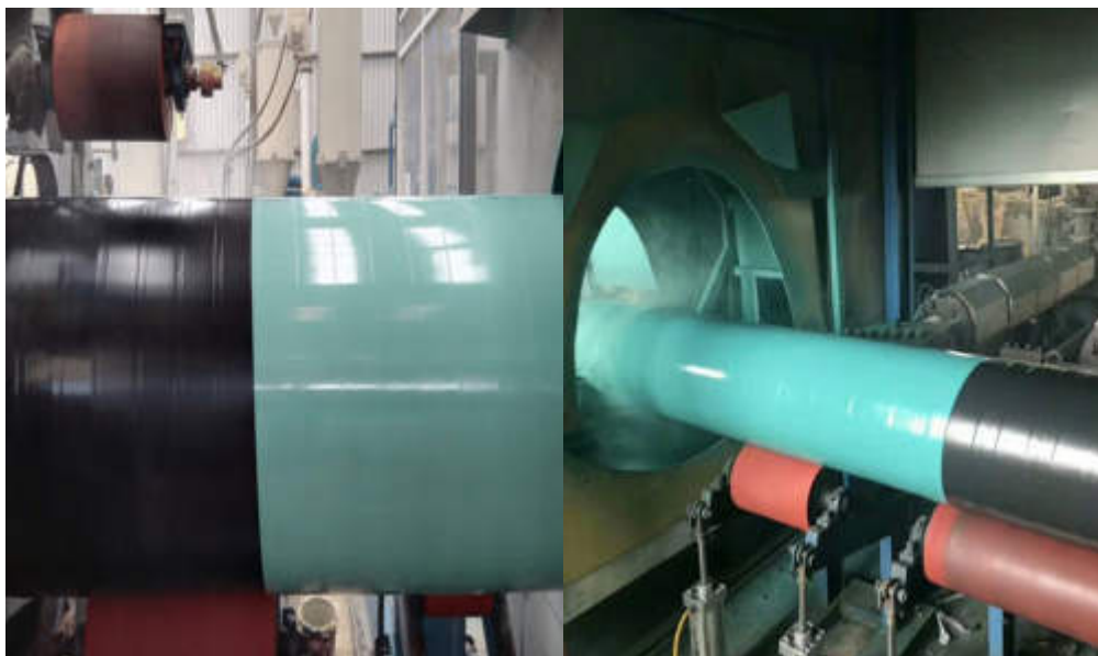
Fig.7.2.9 Adhesive & PE application
