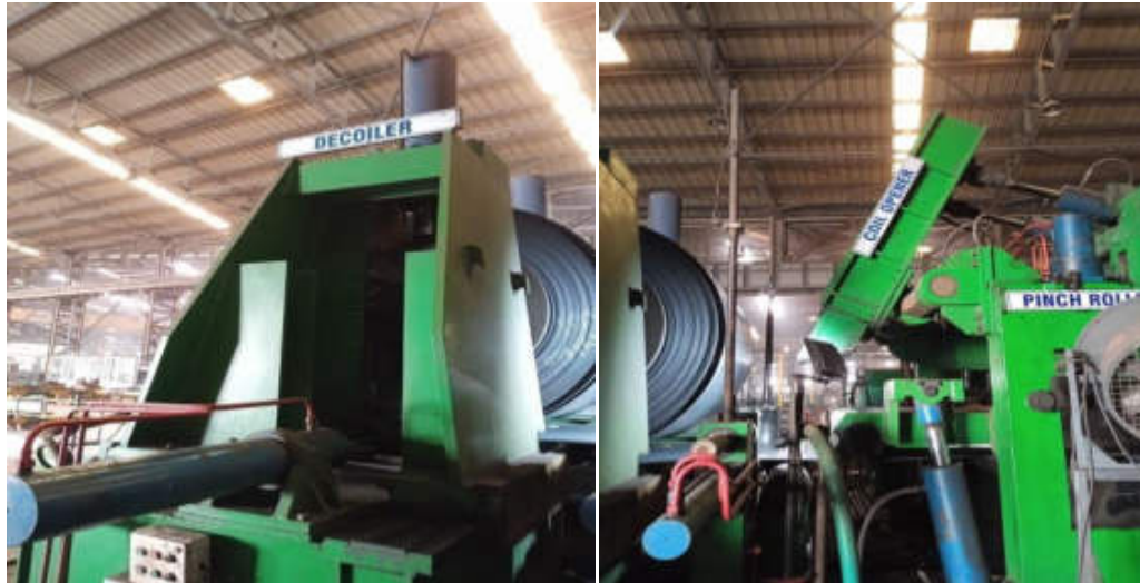
Fig.3.2.1 coil car and un-coiler
