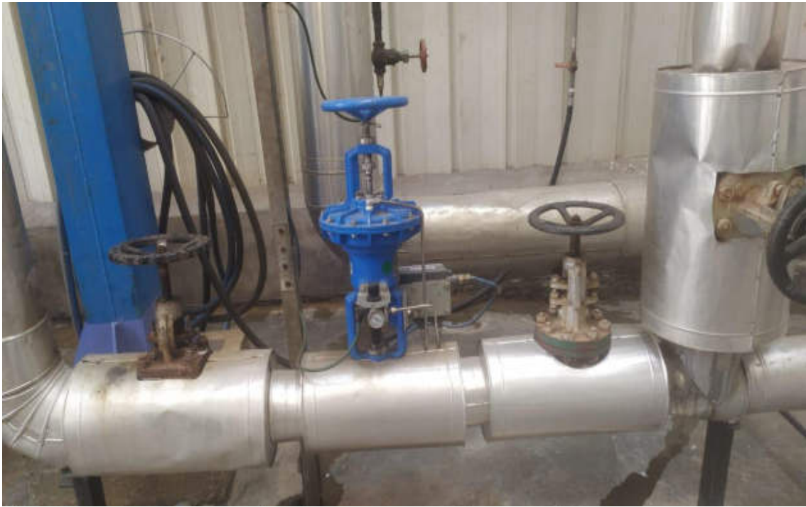
Figure 3.8 Feed Check Valve
