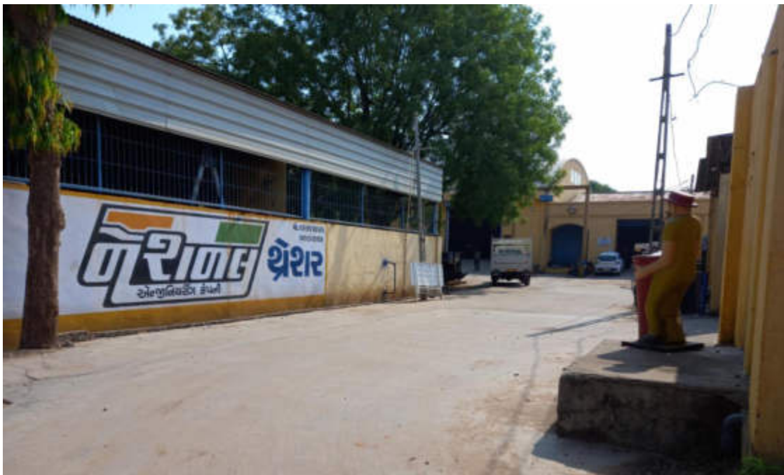
Fig 1.1.1 National Engineering Company
