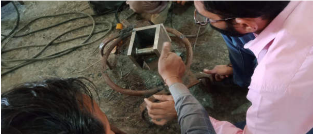
Fig 4.9 Assembly Of Encoder House
