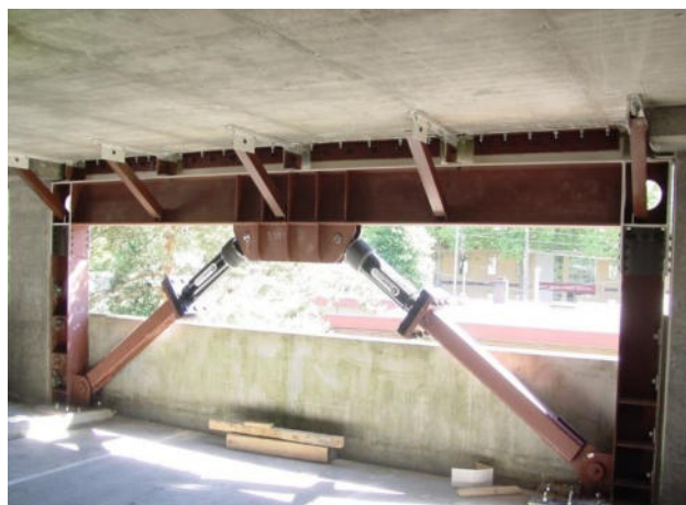
Figure 62 Energy dissipation devices
