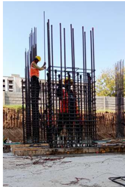
Fig: 6.2 over lapping of column
