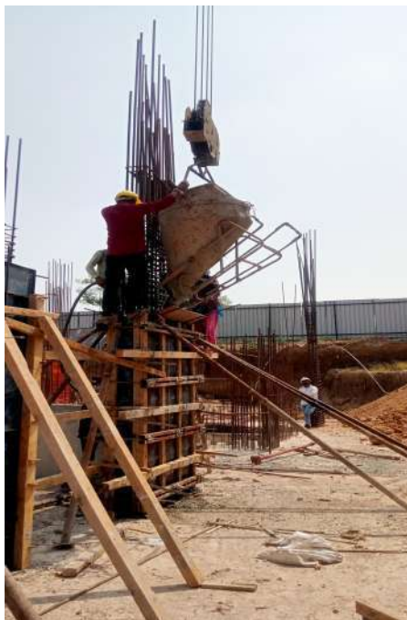
Fig: 12.1 Bucket Concreting
