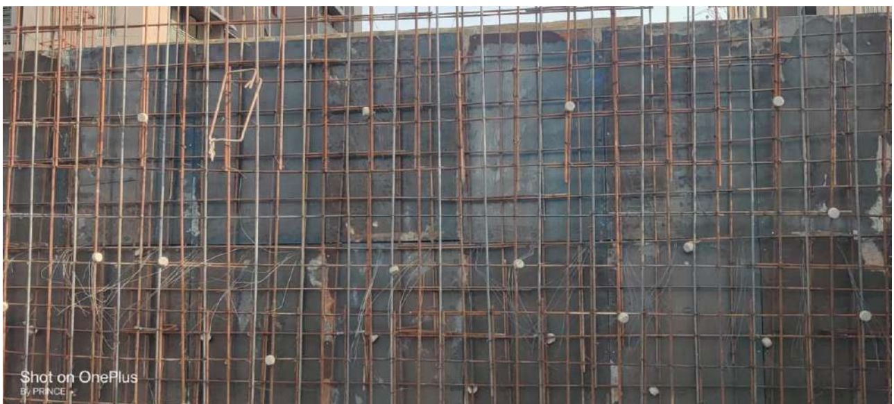
Fig. 8.2 RCC wall steel
