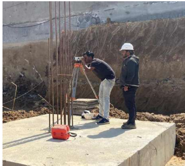
Fig:13.2 Dumpy level check
