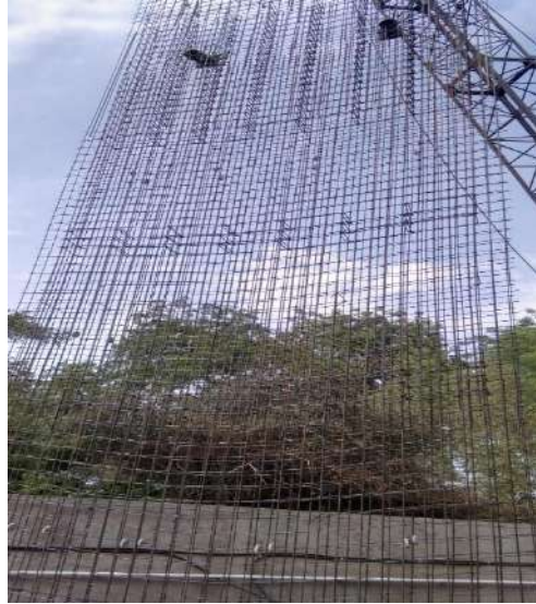
Figure 6: Cage Lifting
