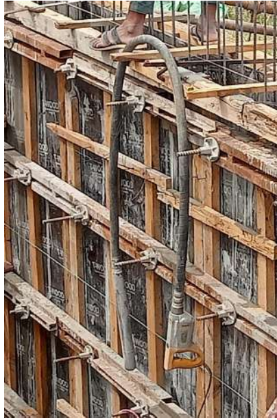
Fig: 13.3 Needle vibrator
