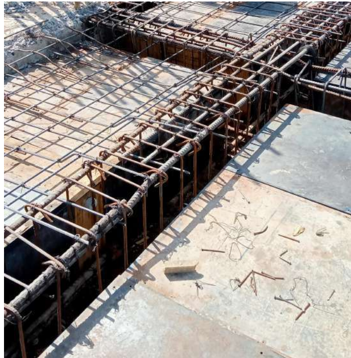
Fig: 2.5 Rectangular beam ( Before casting)
