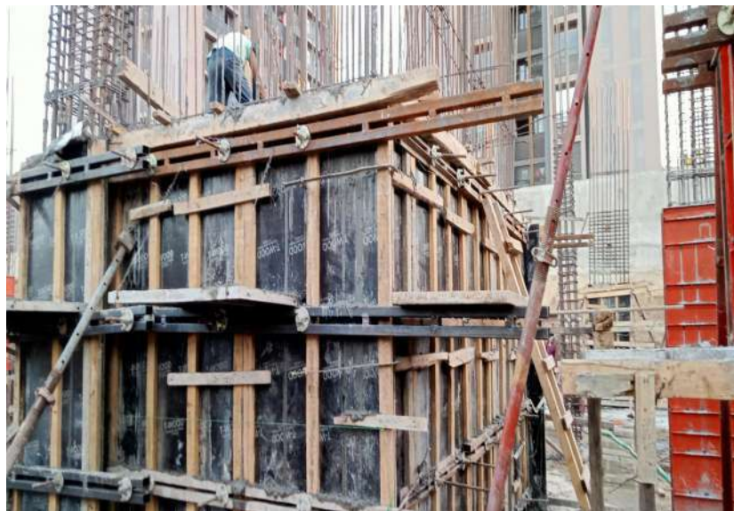
Fig: 9.3 Casting of lift curtain walls
