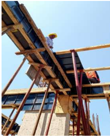
Fig:8.1 Beam Bottom placing
