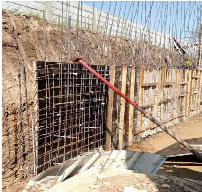
Fig: 2.4 Retaining wall
