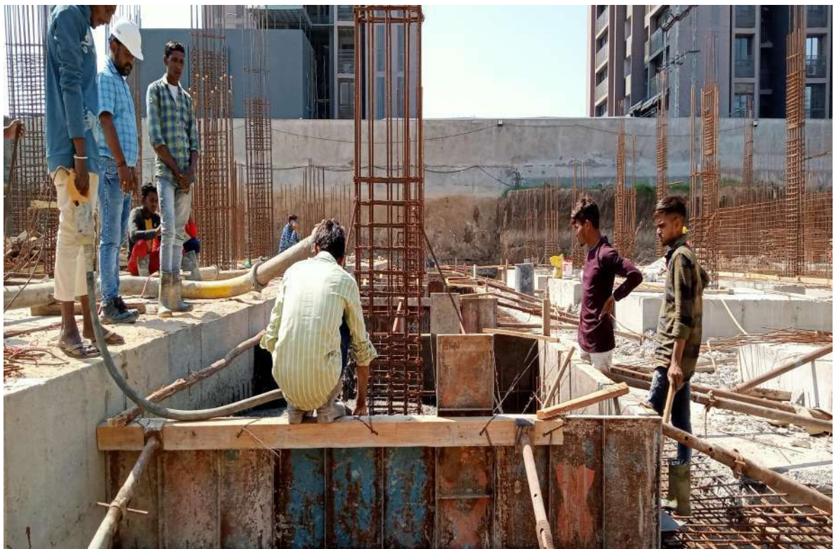
Fig: 5.5 Casting of Footing
