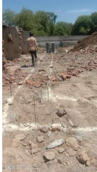
Figure 1: Chuna Line Marking for Construction of Guide Wall
