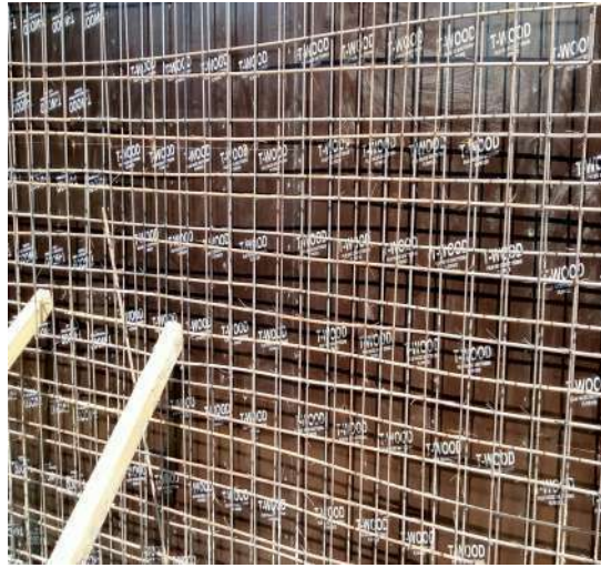
Fig:7.2 Retaining wall steel structure
