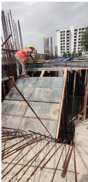
Fig. 7.1 staircase centering
