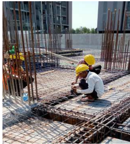
Fig: 8.12 Steel fitting of slab
