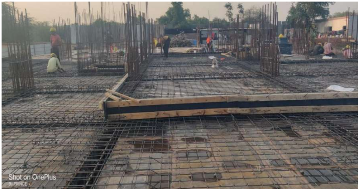
Fig. 9.4 Slab reinforcement
