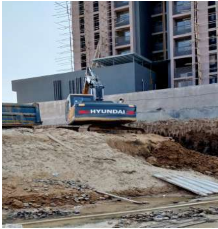
Fig.3.1 Excavation by Back hoe.
