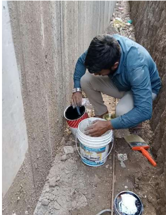
Fig:11.3 Chemical mixing
