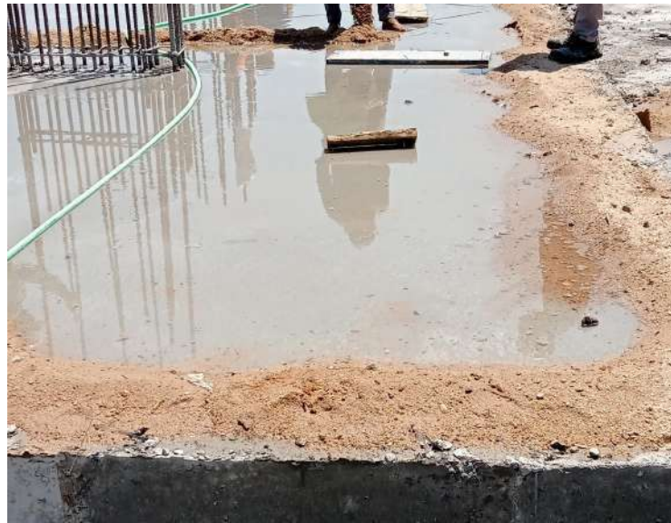
Fig: 14.3 Curing of Slab
