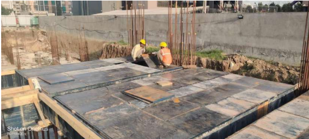
Fig. 9.3 Slab centering
