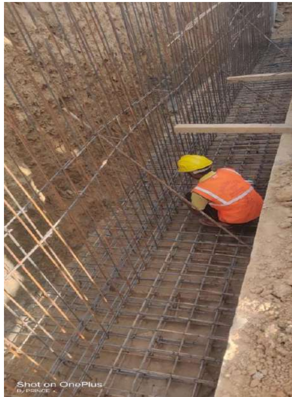
Fig. 8.1 RCC wall steel
