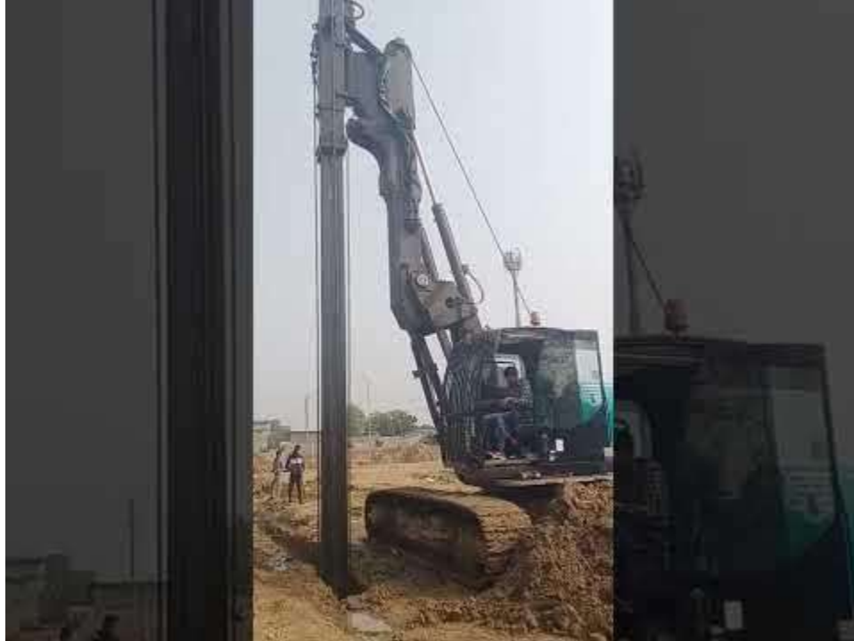
Figure 3: Boring with Casagrande B125 XP Machine
