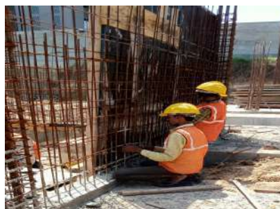
Fig:10.2 Steel fitting of rampwall
