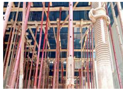
Fig:8.5 Props supporting slab
