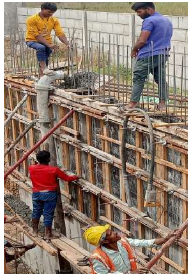
Fig: 7.5 casting of Retaining wall
