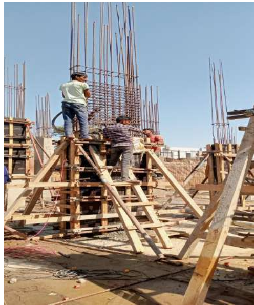
Fig: 6.5 Casting of columns
