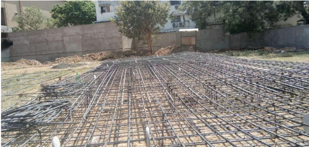
Figure 5: Making of Cage for Panel of Size – 5m
