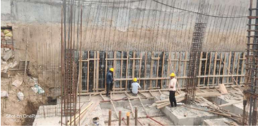
Fig. 8.3 RCC wall shuttering
