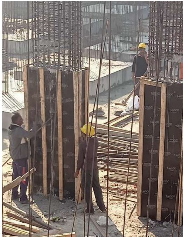
Fig: 6.3 Shuttering of column.
