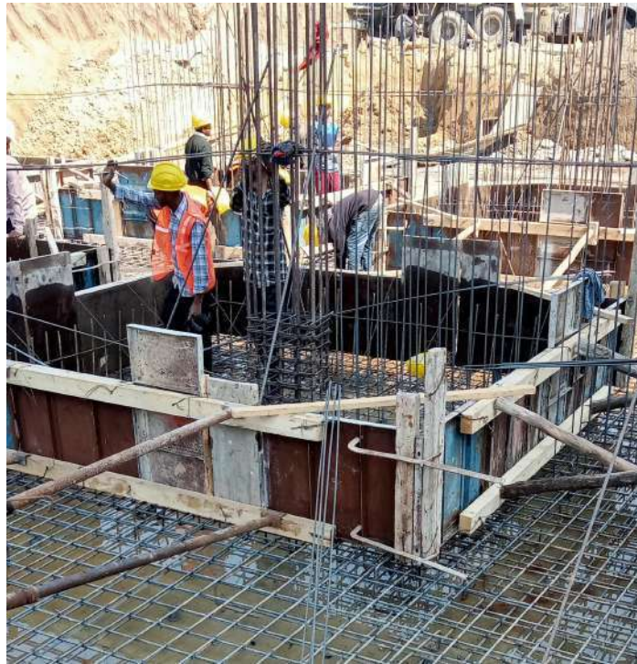
Fig:5.3 Shuttering of Footing
