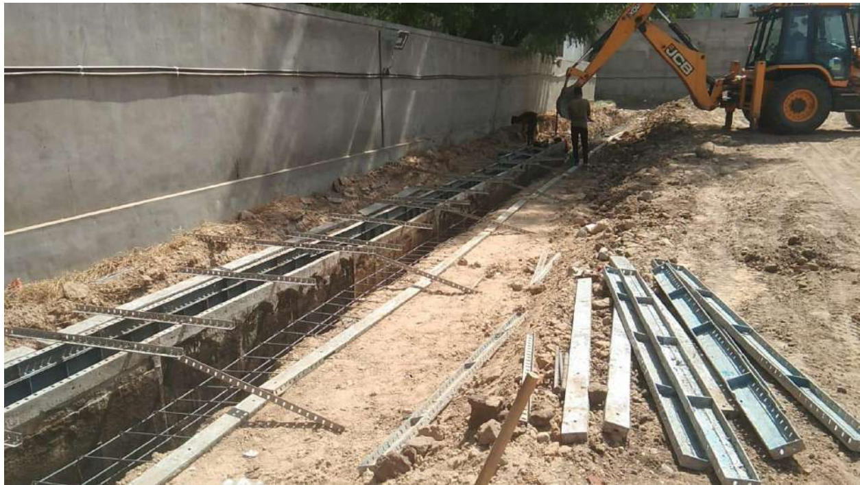
Figure 2: Shuttering Work of Guide Wall
