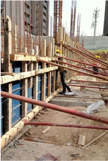
Fig:10.3 Shuttering of ramp wall
