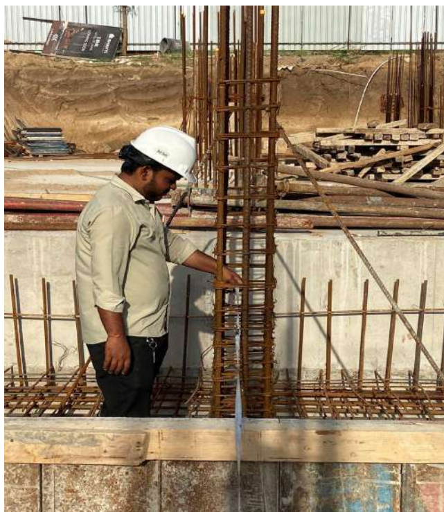
Fig:5.4 Checking of Center of Footing
