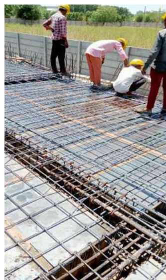
Fig: 8.13 Steel binding
