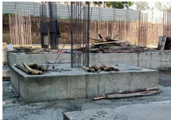
Fig.2.1 Isolated Rectangular footing
