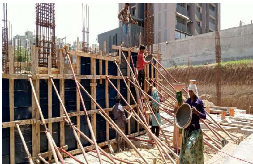
Fig: 10.5 Casting of Rampwall
