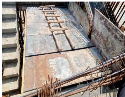
Fig: 8.8 Second stage staircase centering
