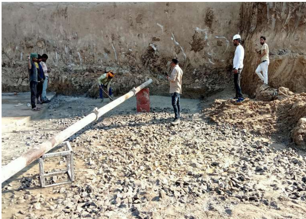
Fig: 4.2 Casting of PCC
