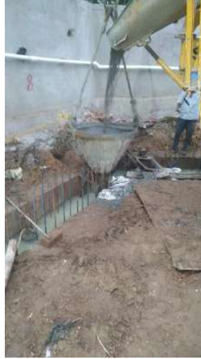
Figure 8: Pouring Panel Using Tremie Pipe
