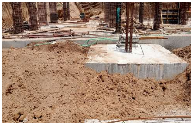
Fig.3.3 Soil filling
