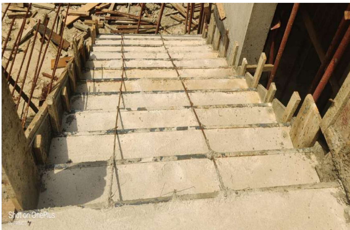
Fig. 7.4 staircase casted
