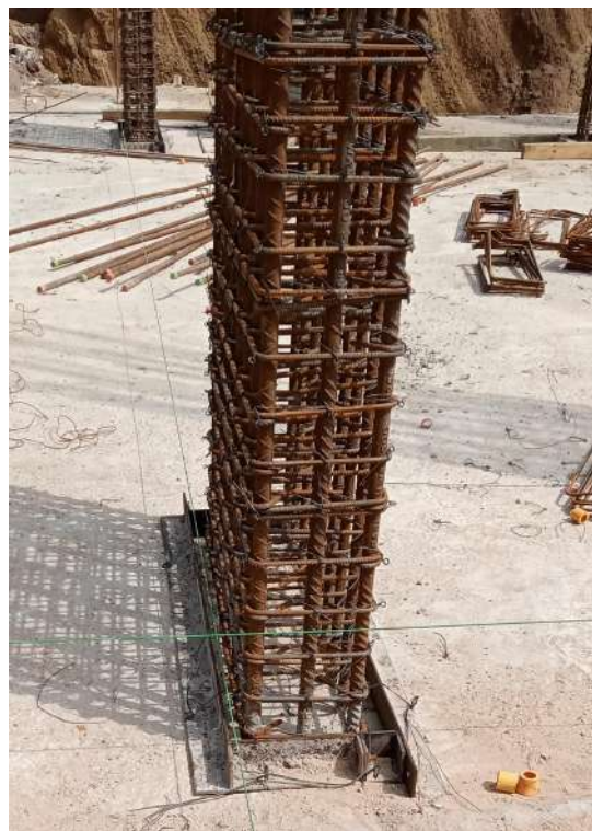
Fig: 6.4 Starter shuttering,line dori
