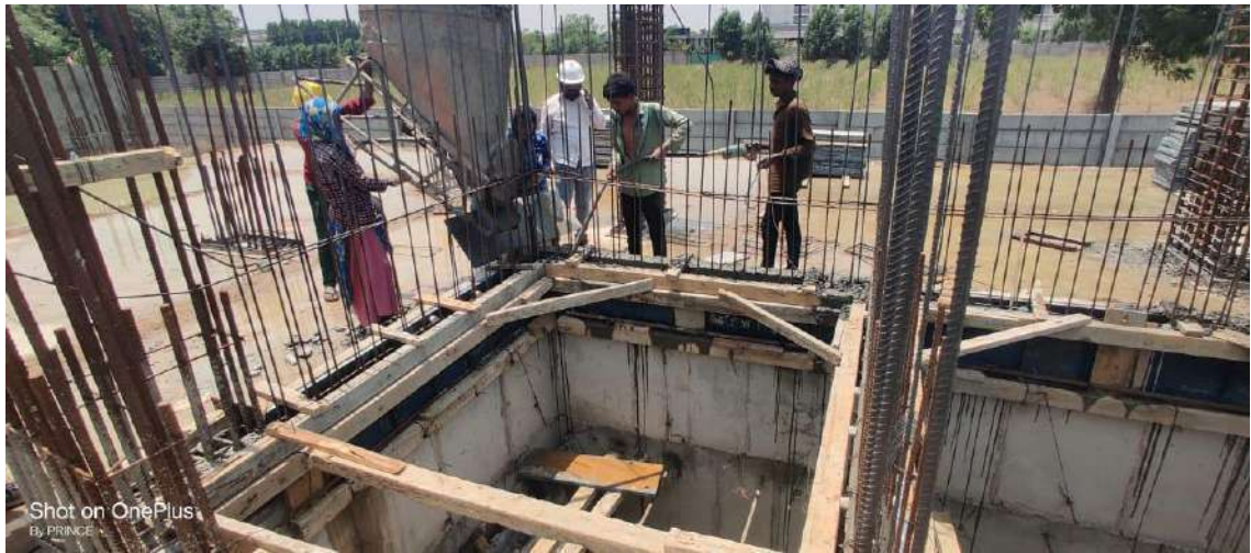
Fig. 6.3 Lift casting
