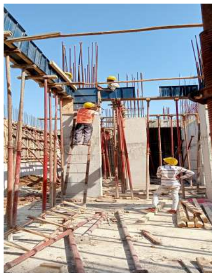
Fig:8.3 Beam Side shuttering
