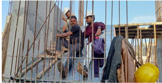
Fig: 8.7 Centring of Staircase
