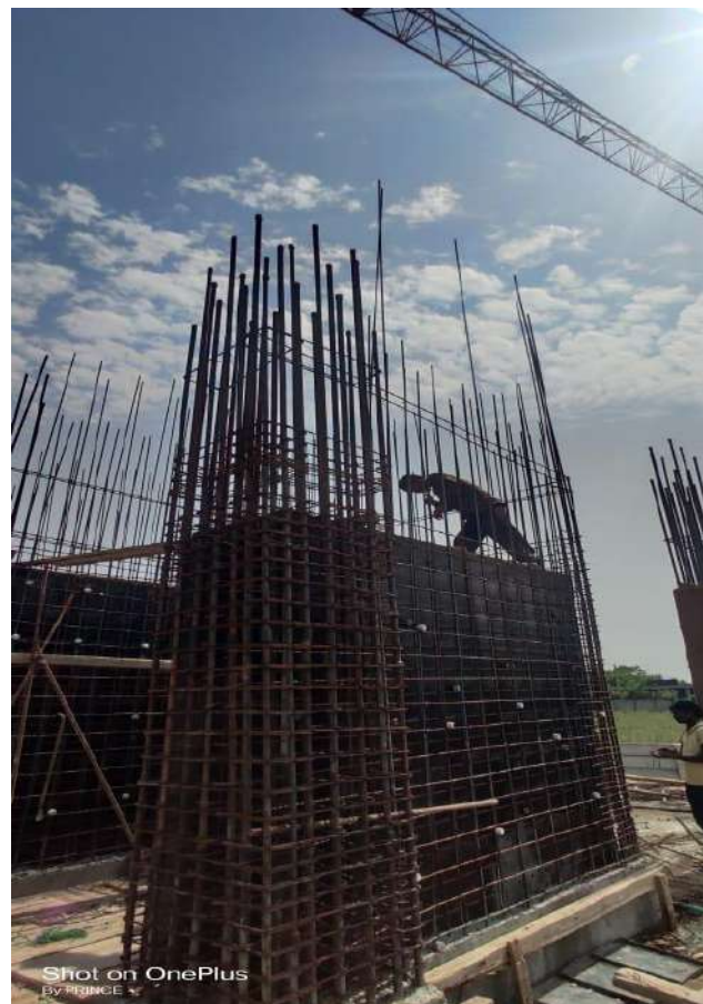
Fig. 6.1 Lift steel
