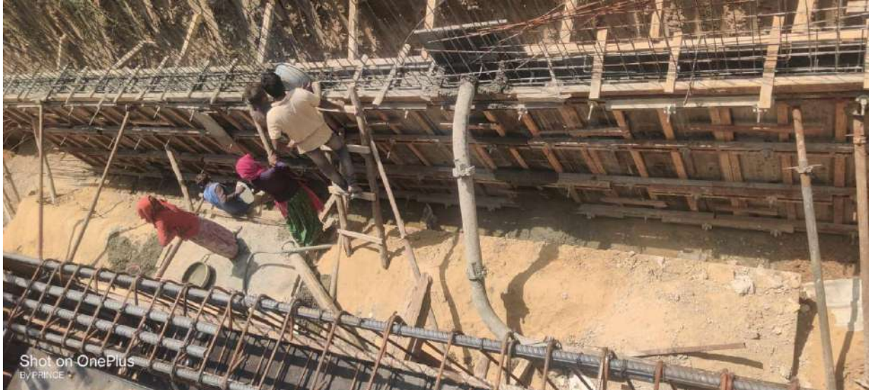
Fig. 8.4 RCC wall casting
