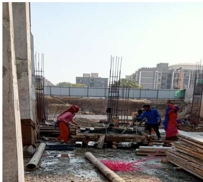
Fig: 6.6 Concrete pumped on platform
