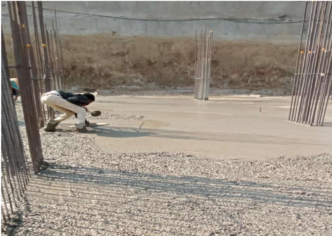
Fig: 5.6 Finishing of Raft footing
