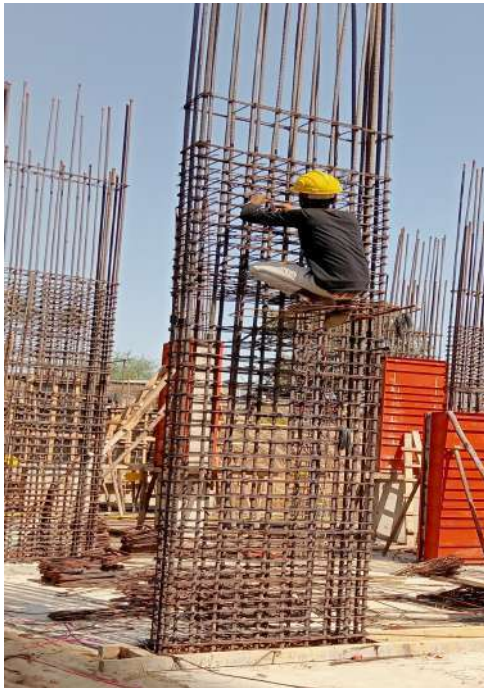
Fig: 6.1 Steel fitting of Column
