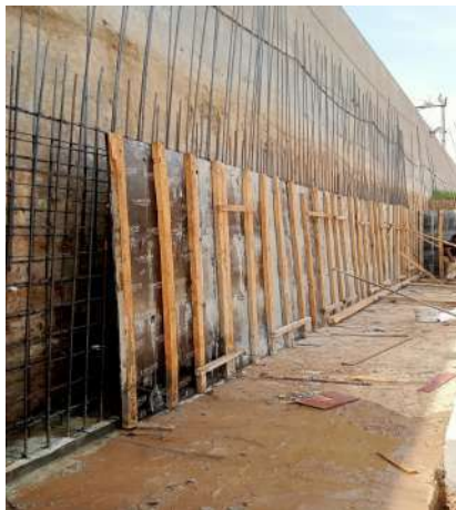
Fig:7.3 Single side shuttering
