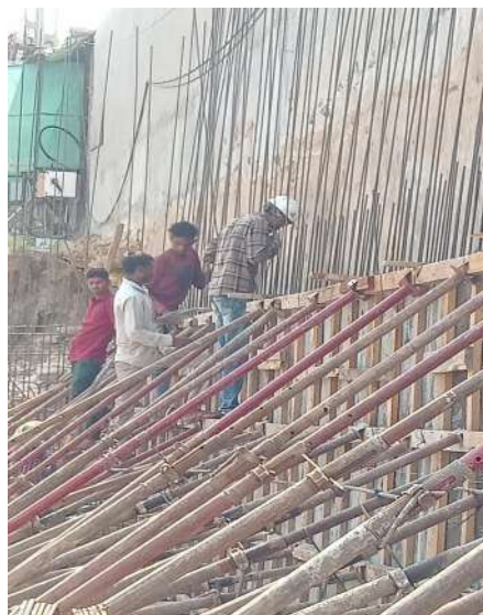
Fig: 7.6 One sided shuttering Retaining wall
