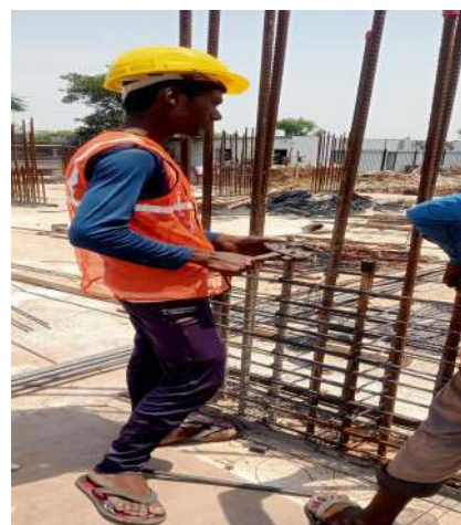
Fig: 14.7 Coupler placing
