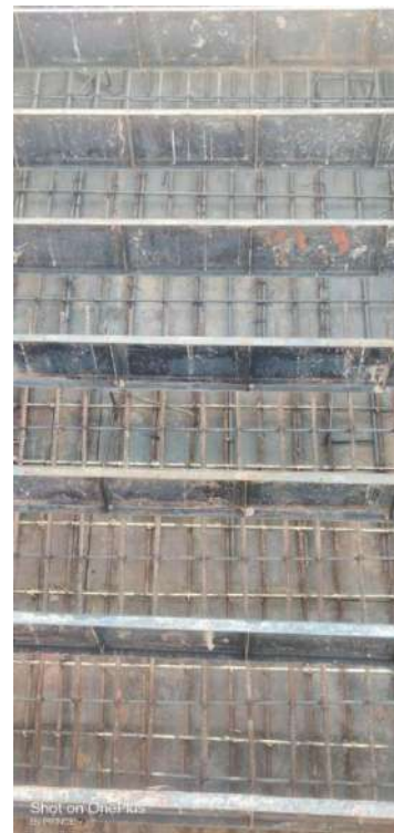
Fig. 7.2 staircase centering & steel
