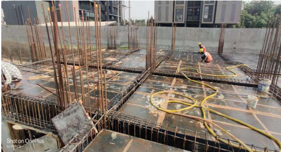
Fig. 9.4 Beam reinforcement
