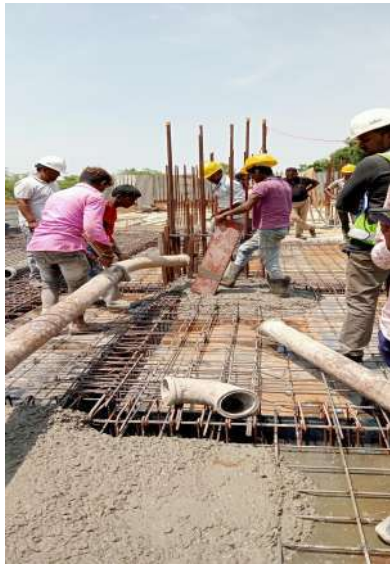
Fig:8.14 Concrete placing
