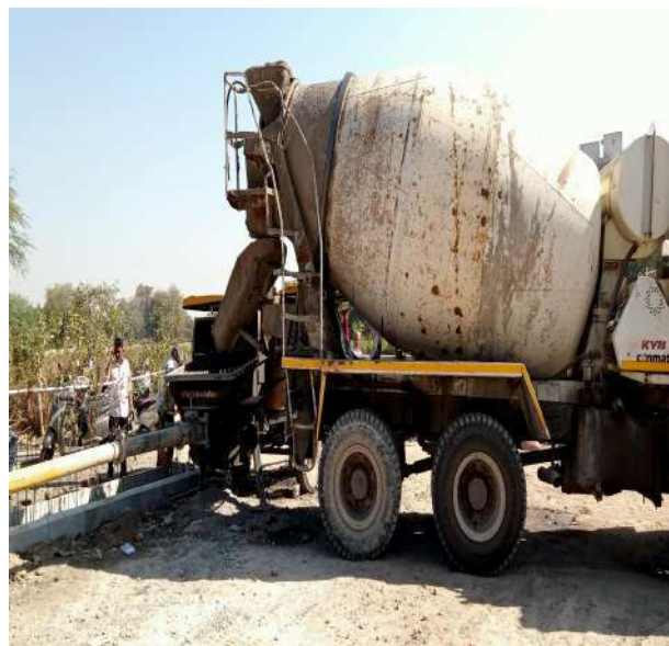
Fig: 12.2 Hopper and RMC truck.
