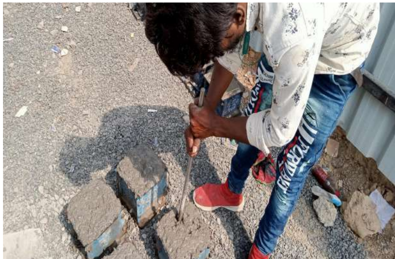
Fig:12.4 Compacting of Concrete
