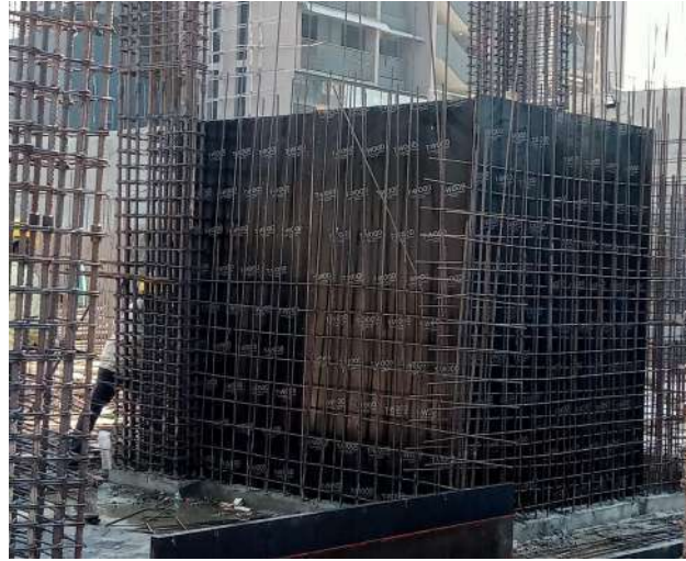
Fig: 9.2 Shuttering of lift
