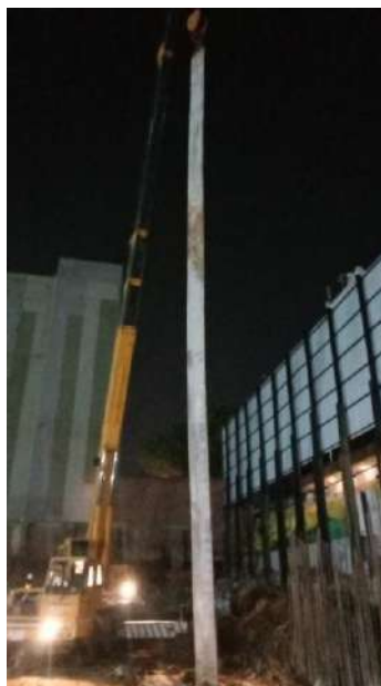
Figure 7: Stop End Lifting & Resting
