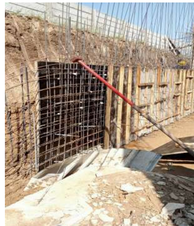
Fig:7.4 Double side shuttering
