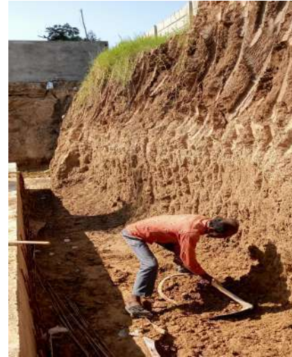
Fig.3.2 Manual excavation
