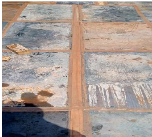
Fig:8.6 Tap in sheet joint
