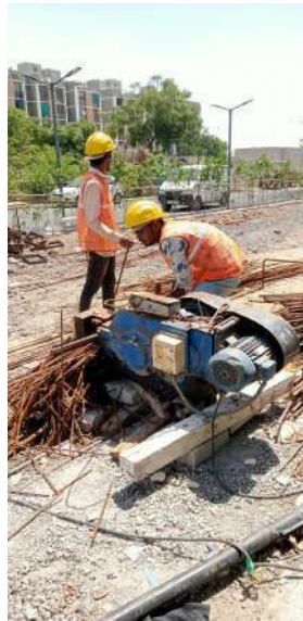
Fig:5.1 Steel Cutting
