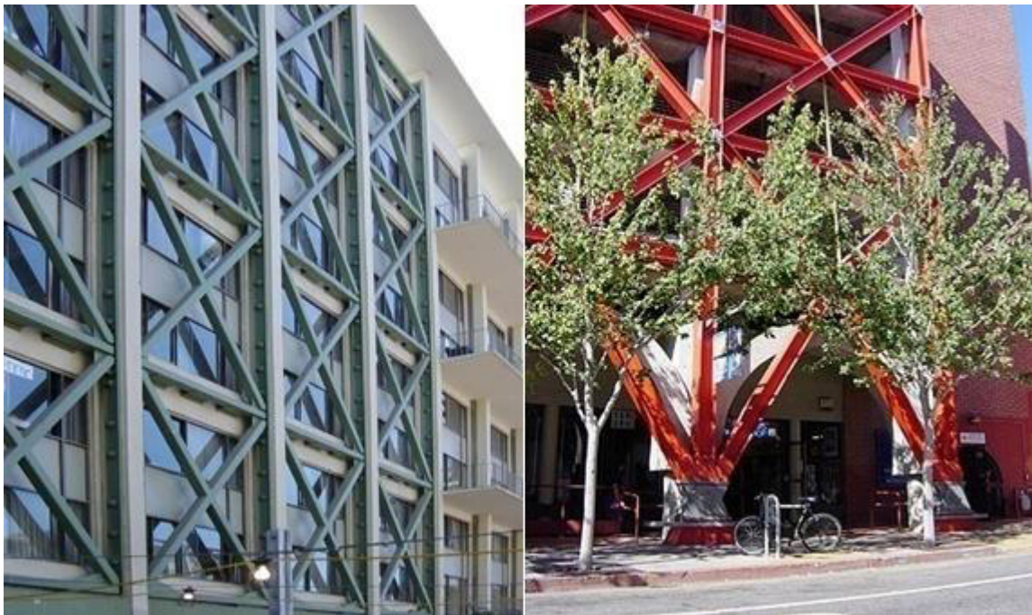
Figure 64 Infill shear trusses
