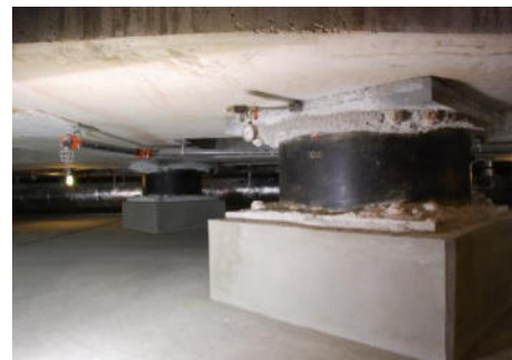
Figure 61 Base isolation
