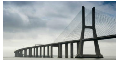
Figure 65 High performance concrete
